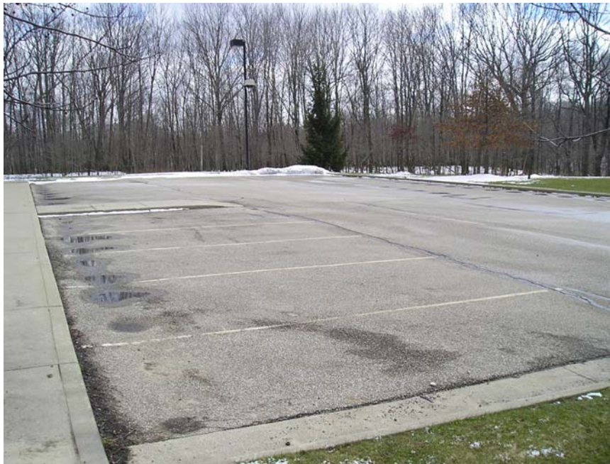
Photo 6: Building parking area section
