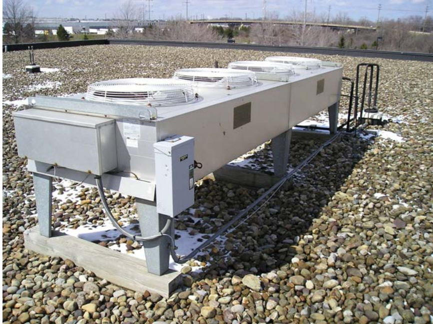
Photo 1: General roof area
