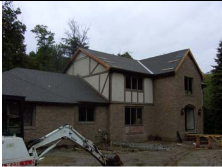
Figure 2 – Work in Progress
