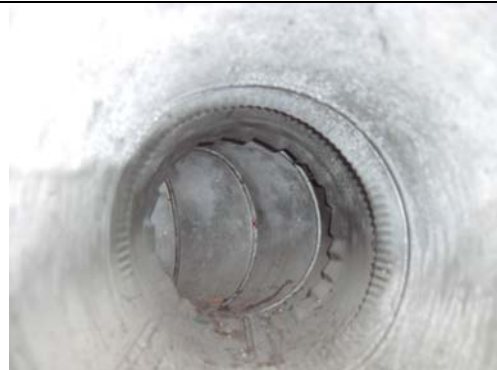
Figure 5 – Ductwork (New Construction)
