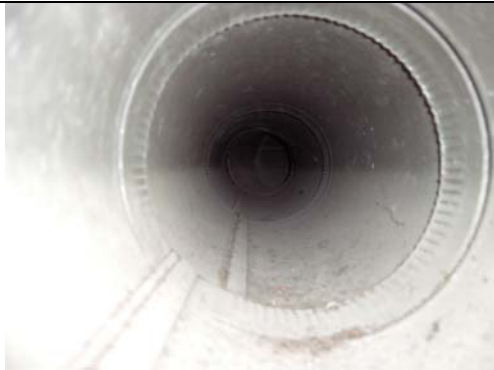
Figure 4 – Ductwork (New Construction)
