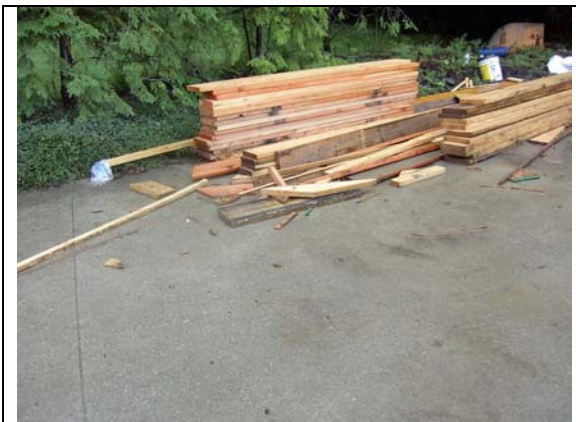
Figure 1 – Materials Stored On Site
