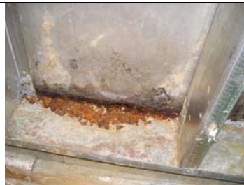
Figure 3 Inside exterior wall cavity
